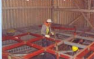
Reinforcing the observatory floor
